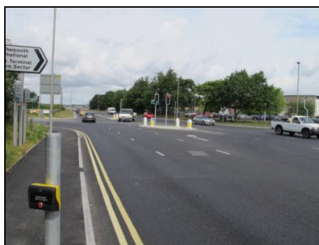
Figure 3: Parley Lane Airport Access Junction
