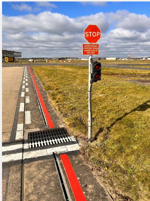
ATC and Fire Station LVP warning signs
