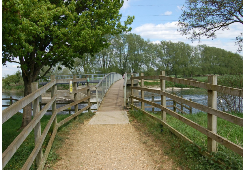
Sustrans Connect 2 Scheme – The narrow bridge at Throop
